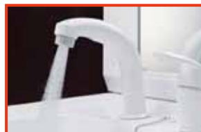
Upgrading to Water-Efficient Equipment (Joy Oyamadai)
