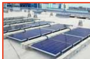
Installation of solar panels (Gran Casa Saitama Shin-toshin)
