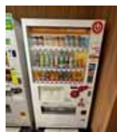
Installation of donation-type vending machines (Daiwa Tsukishima)
