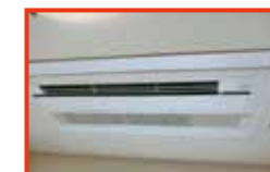
Implementation of air conditioner replacement (Good Time Living Amagasaki Eki-mae)
