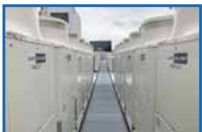
Upgrading of air-conditioning equipment (Daiwa Ginza)
