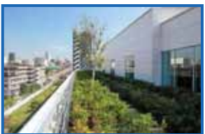
Installation of rooftop garden (Daiwa Azabu Terrace)
