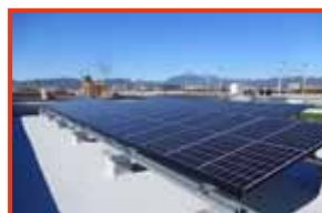
Installation of solar panels (Gran Casa Kyoto Eki-mae)
