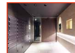
Installation of delivery boxes (Gran Casa Higashi-nakano)
