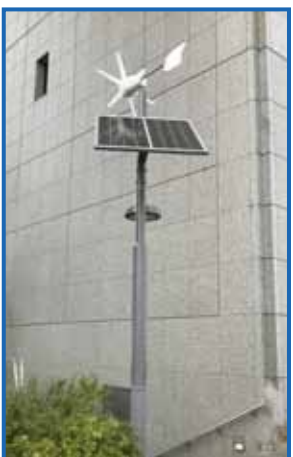
Installation of Solar-Wind Streetlights (Daiwa River Gate)
